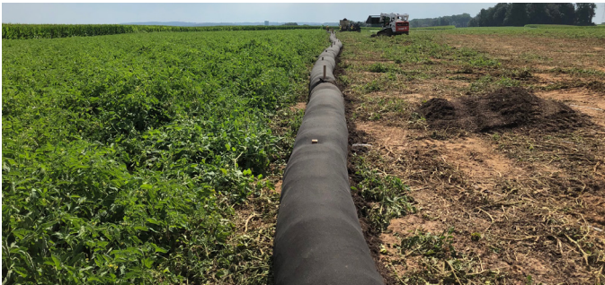
Filter sock used as perimeter protection on a pipeline project.
